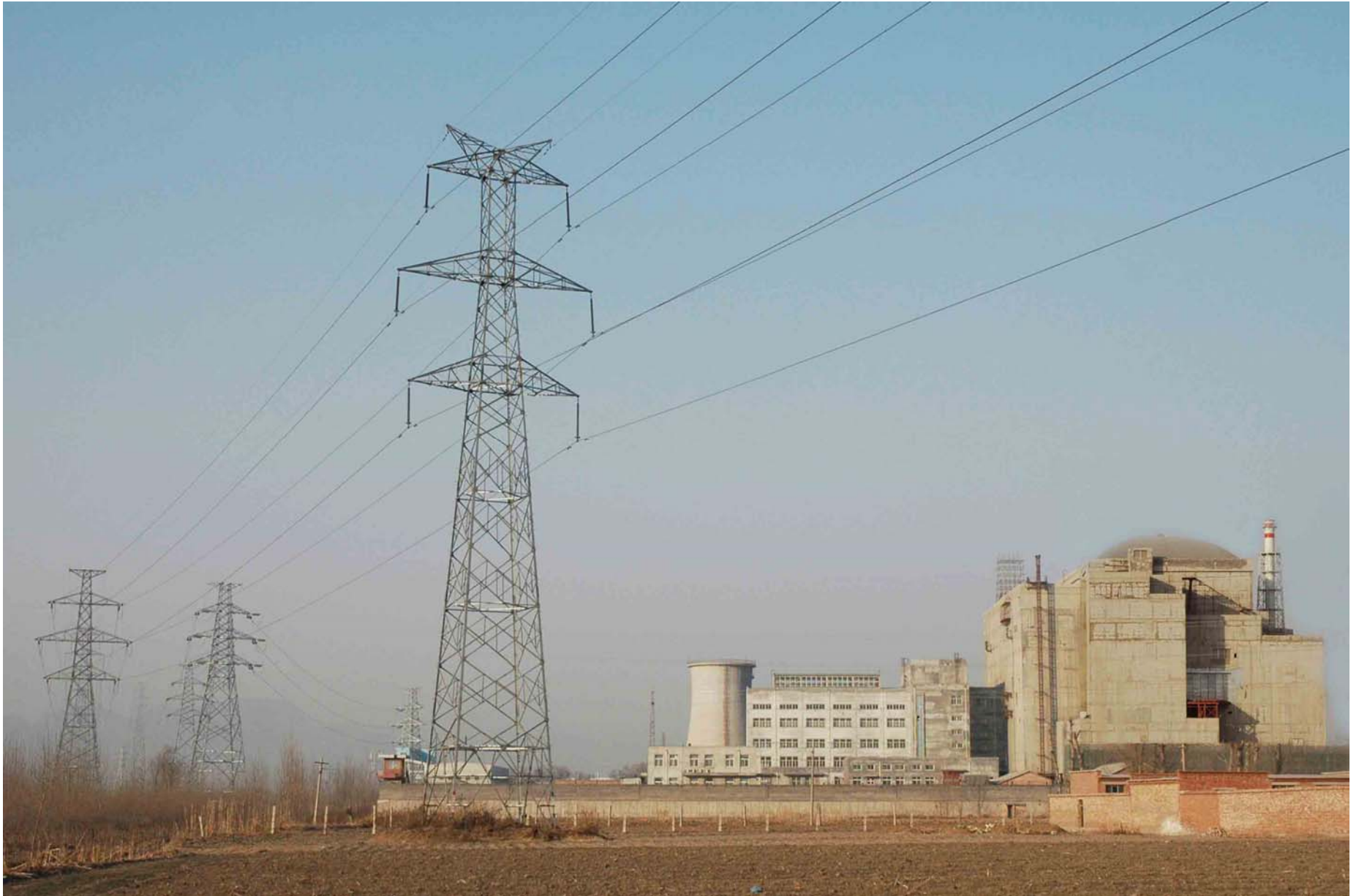
National Grid comes to the site (2007.01.28)
